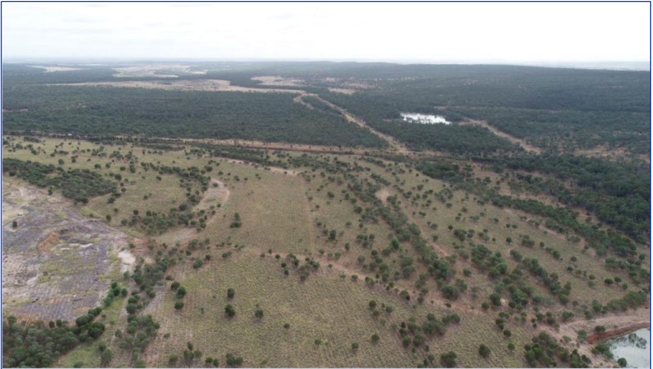
Figure 1-7 Existing rehabilitation at Y Pit (ML70049)
