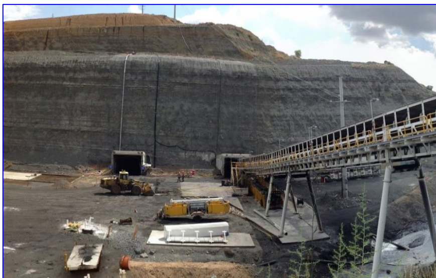
Figure 5-11 Entrances to the existing Ensham underground mine.
