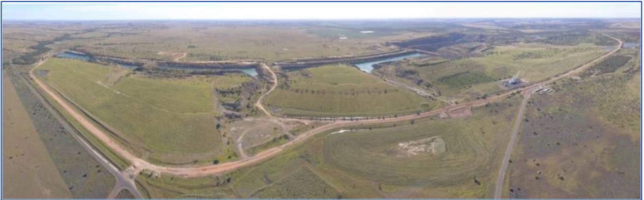
Figure 1-5 Existing rehabilitation at AB Pit (ML7459)
